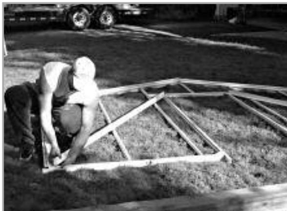
5. Install the polybar on each side of the door frame (*make sure that the angle cut on top matches the slope of the roof*).
