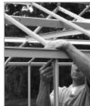
*At this time fasten the greenhouse base/sill to the foundation.*
