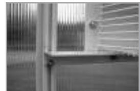
NOTE: When installing fan into Triple Wall Greenhouse, tape the edges with aluminum foil tape.
