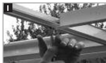
11. Your greenhouse is now ready for putting on the 1/8" foam strips. Do not put the foam strips on the base or beside the door. Only use the foam on the poly bars. Do not put foam strips on the gutter (See Page 26).
