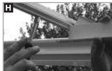
**NOTE:** Fasten the greenhouse base/sill to the foundation using #8 x 1" screws (if it is on concrete, drill holes using a concrete bit and push the plastic plugs into the holes). If possible, lift the greenhouse and seal below the base before fastening the greenhouse to the foundation.
