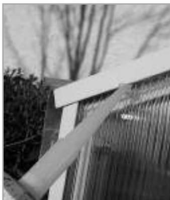
6. Wherever the polycarbonate sheets are sitting in a track or aluminum "H", seal the edge, including the end poly bars. Also seal the inside of the sidewalls because greenhouse humidity runs along the walls and into the bottom track.
