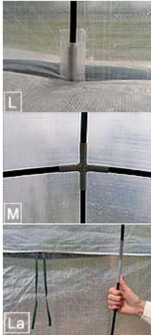
**Step 10:** Beginning with **one** of the L-shaped fiberpoles, insert the capped end into the pocket in the center near the floor. (See "L"). Insert the uncapped end into the X-shaped piece. (See "M"). While assembling the L-shaped pole, keep it to one side. This will relieve some tension and allow for easier assembly. (See "La").
