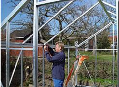
The roof profiles are assembled.
