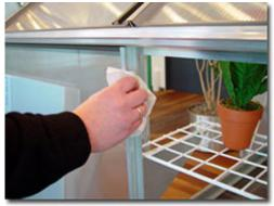
The frame is degreased with acetone, The polycarbonate sheets only have to get the best fitting.
