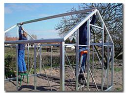
Now assemble the ridge. Loosen the bolts in the top of the gable, to make assembly easier.
