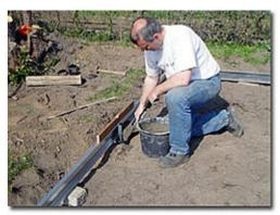
Pour the concrete into the holes and let it harden for 24 hours.
