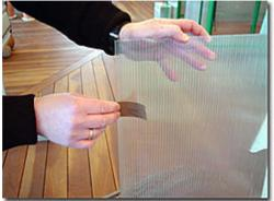
Sand the edge of the polycarbonate until you have installed it. Otherwise it sheets, to make the silicone seat more onto the frame. (Only in areas where effectively once it its glued.
