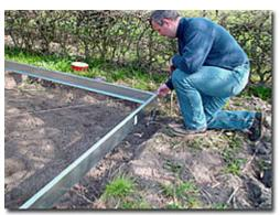
measurement must be the same for both diagonal measurements. This ensures that the base is square.
