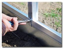
If you bought a Juliana steel base, you must fasten the greenhouse to the assembled lift them up onto the base. base using j-plates. The small bow are pushed under the base and fastened to the greenhouse bolt through the long hole.
