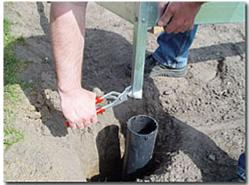
Before you put the ground anchors into the pipes you have to splay them. measurements again to ensure that
