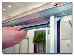
The A gaskets are installed into the top of the section as shown. The "flap" bottom of the sections in the same of the list is pushed into the profile in way. the top.
