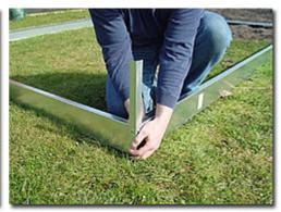
The ground anchors are used to fix the sides and ends together.
