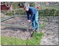
Place a stick through every ground anchor so that you know where to dig the holes, and remove the base.
