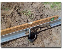
Level the base and check the diagonal the base is level and square.
