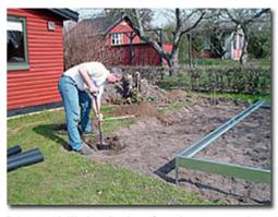
Dig or drill the holes for the ground anchors to be connected to the ground. The holes should be at least 32 inches deep, so that the base is fitted to frost free depth.
